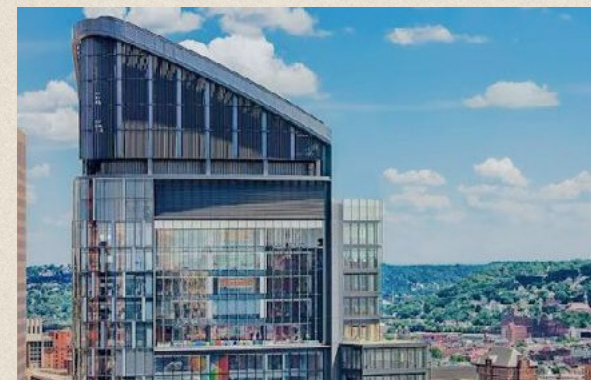
THE TOWER AT PNC PLAZA, PITTSBURGH
